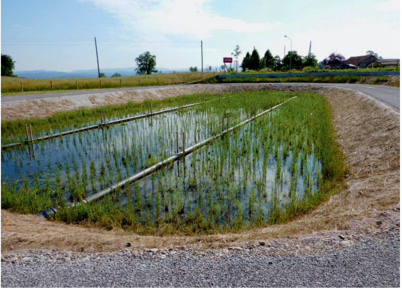
2 | SABA Chringelbach, Forchstrasse (Foto: ilu AG). 2 | SETEC de Chringelbach, Forchstrasse (photo: ilu AG).
