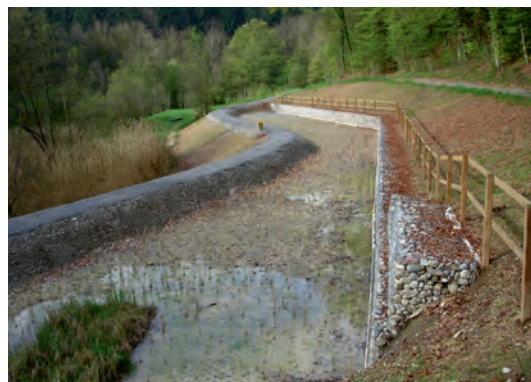
Abb. 2 A20.1.4: SABA Wüerital, Sandfilter, Bau 2007.
